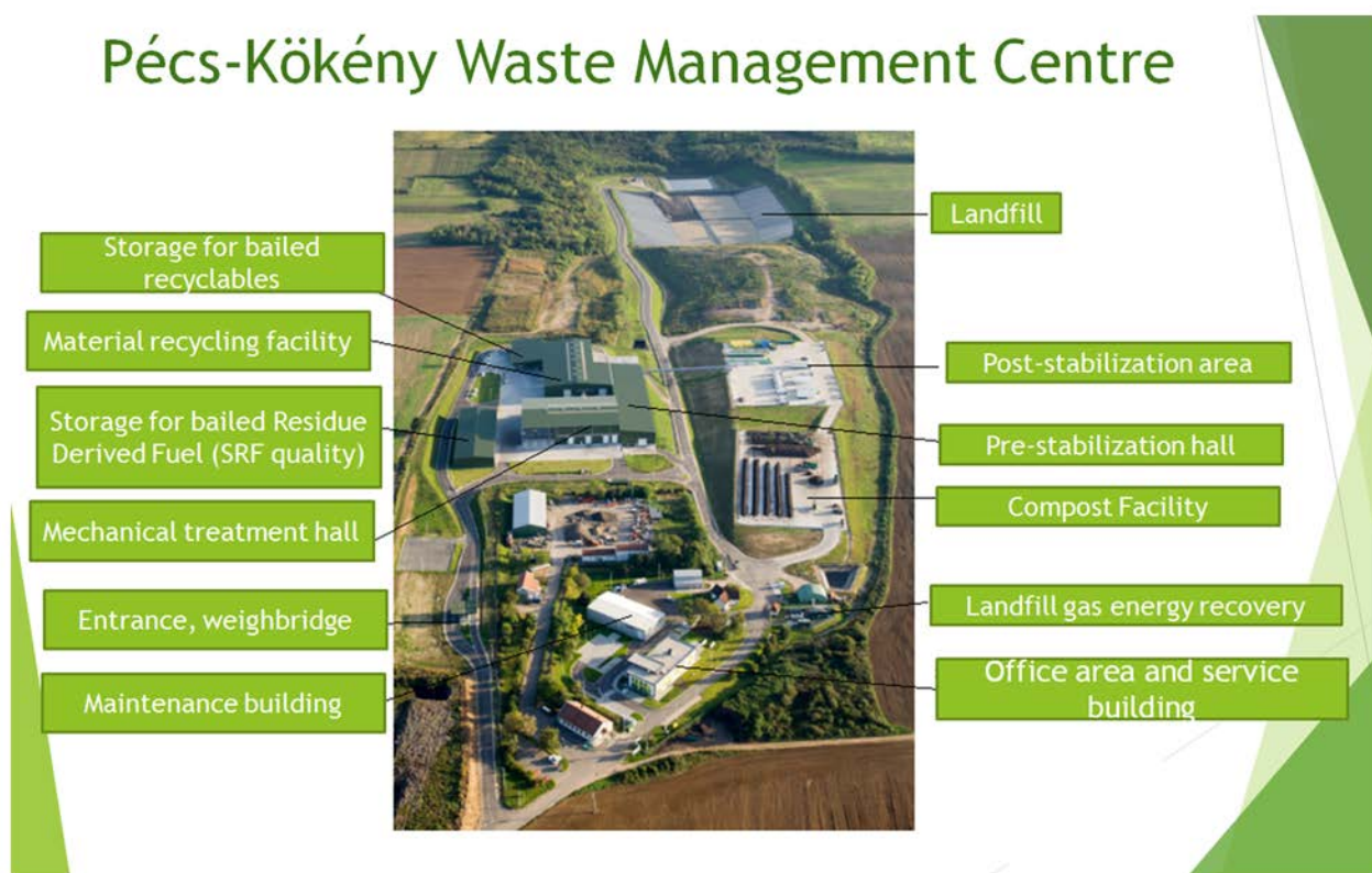
Figure 2: Construction of the Kökény Waste Management Centre
