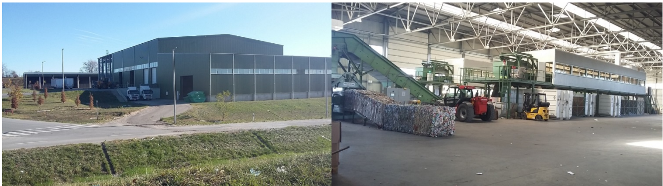
Figure 4: The Mechanical-biological Waste Treatment Plant of Kökény
